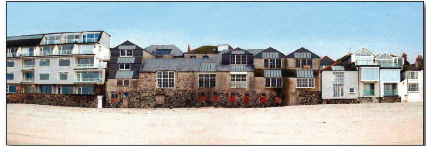
Above: Porthmeor Studios and Fish Lofts with Improvements
